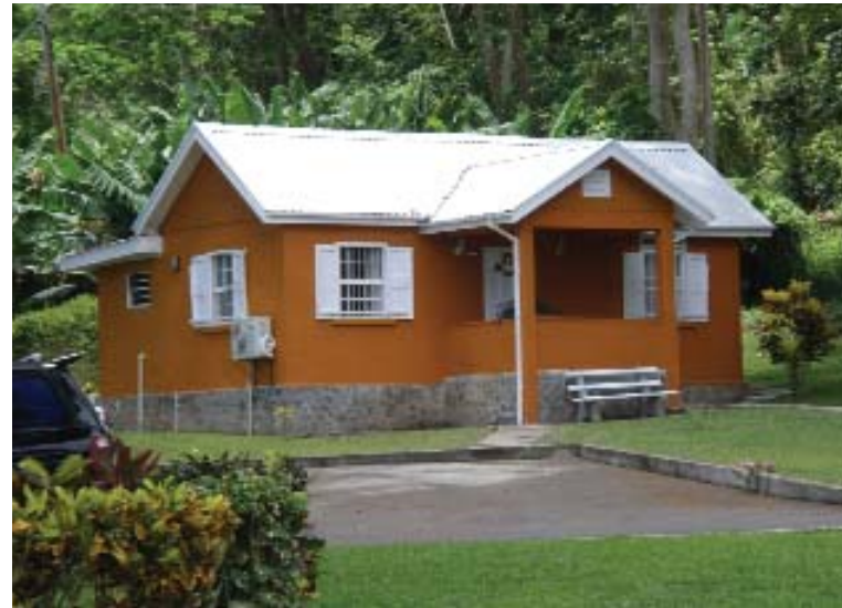
Refurbished cottage, Open Campus, Dominica
